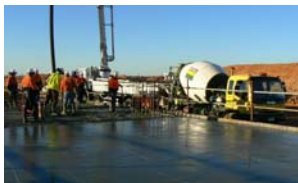
Boddington Gold Mine (Concrete), WA
