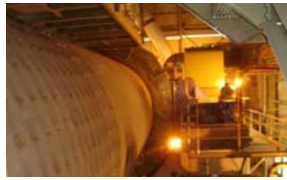
Berrima Cement Mill 7 Upgrade
