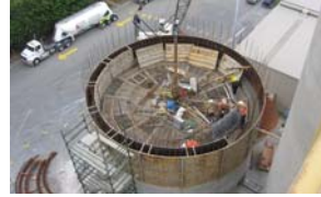
Sunstate Cement Capacity Upgrade
