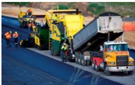
Construction of EastLink, Melbourne
