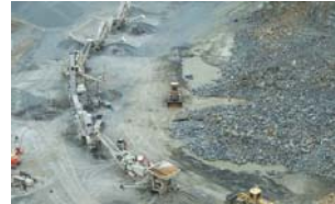
Mobile Crushing Rig, Queensland
