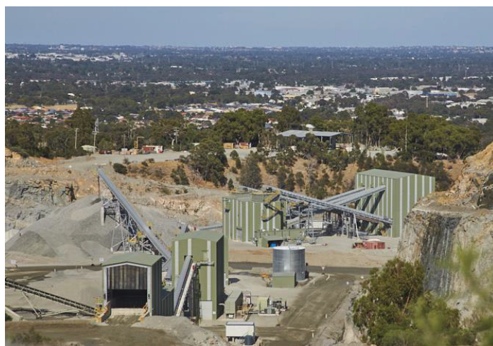
Boral Australia, plant upgrade at Orange Grove Quarry, WA
