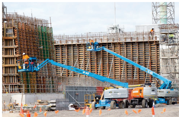
Construction of Boral Australia's clinker grinding facility, Port of Geelong, Vic
