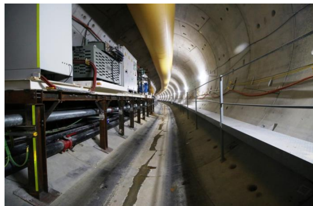
Forrestfield Airport Link, WA (Photo supplied courtesy of Salini)
