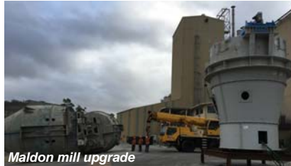
Maldon mill upgrade
