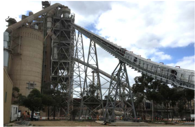
Resource derived fuels loader for the Berrima Kiln
