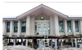
House lift with foundation products
