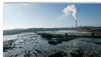
Fly ash pond at operational facility
