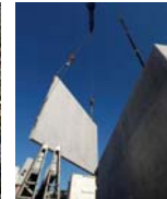
PRECAST concrete panels
