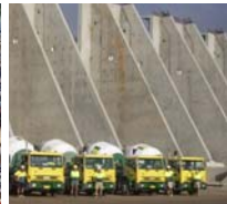
CONCRETE for the Port Botany Redevelopment NSW
