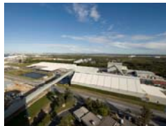
Pinkenba PLASTERBOARD plant, QLD
