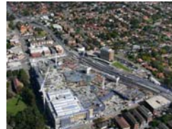
CONCRETE PLACING, Shopping Centre NSW
