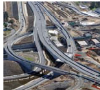
ASPHALT for the SAFElink project QLD
