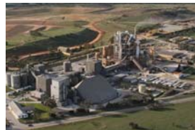
Blue Circle's Waurn Ponds CEMENT works
