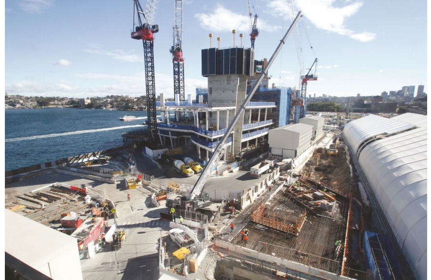
Boral supplying Envisia concrete to Crown Sydney Barangaroo, NSW 1
