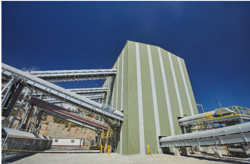
Plant upgrade at Orange Grove Quarry, WA
