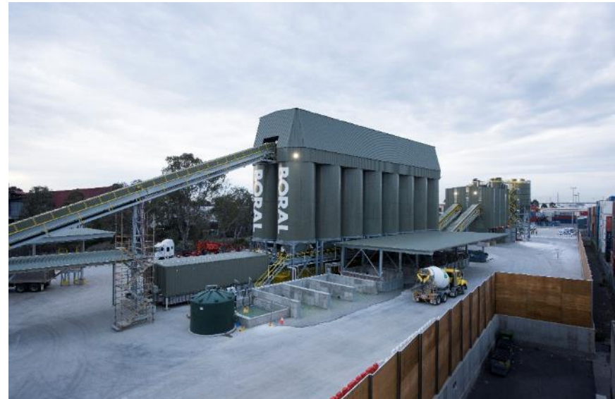
New West Melbourne Concrete Plant, Vic
