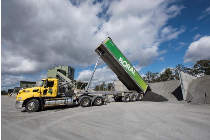
Redbank Plains concrete batch plant, Qld
