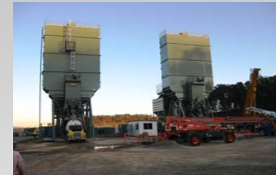
Contracts awarded for supply of concrete to Curtis Island LNG and Gladstone LNG projects in Qld.
