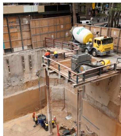
Boral delivering concrete to a Sydney commercial building project
