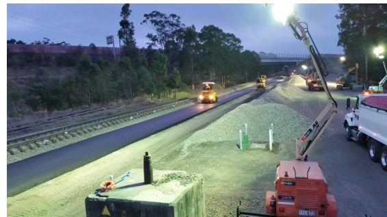
Figure 5 completed 2 nd asphalt layer with ballasted track adjacent
