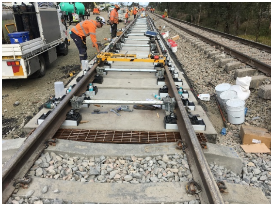
Figure 22: Final track adjustment with RhoFAS and HERGIE prior to grout pouring
