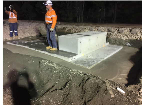
Figure 16: Insitu grout pouring
