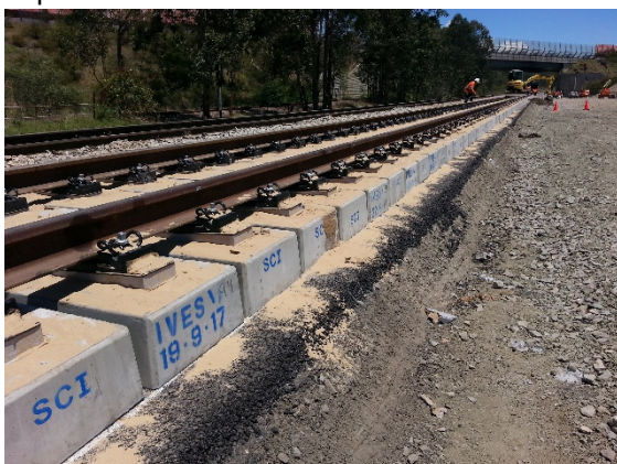
Figure 25: Asphalt layer with sufficient shoulder width
