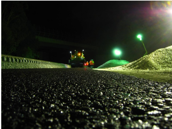
Figure 6: Condition of asphalt layer
