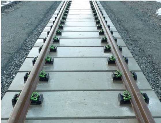
Figure 2: Non-ballasted track IVES
