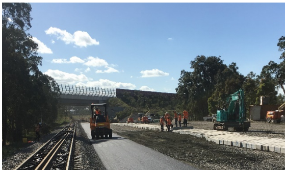
Figure 24: Asphalt layer suitable for road traffic during construction period
