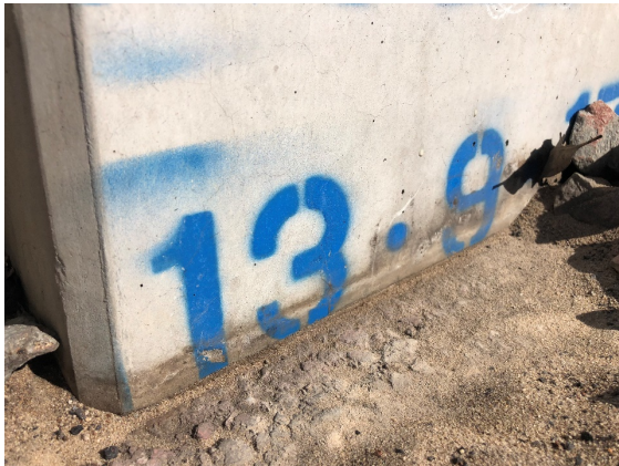
Figure 32: Railpave layer under IVES
