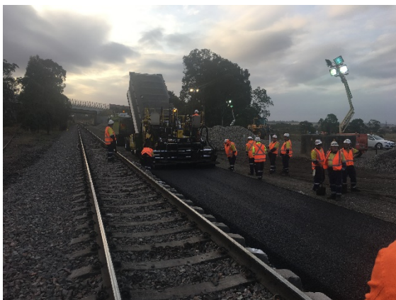
Figure 19: Placement 1st asphalt layer RailPAVE with road finisher
