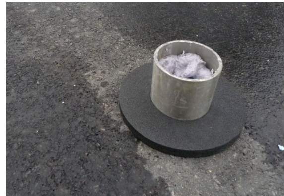
Figure 29: Dowel connection placed in asphalt layer
