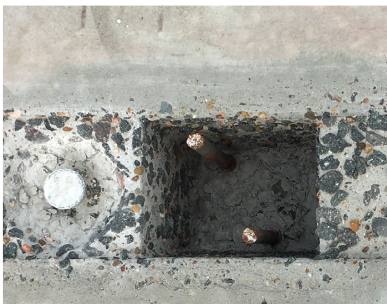
Figure 27: IVES pockets with roughened surface for optimised bonding characteristics
