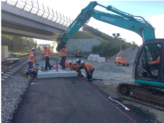
Figure 21: Placement of IVES elements
