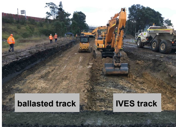
Figure 14: Excavation for double track reconditioning works
