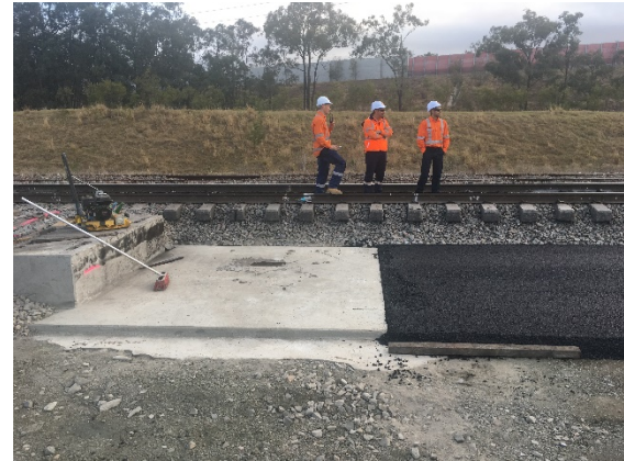
Figure 20: Asphalt layer joining pre-cast VTRAS abutment elements
