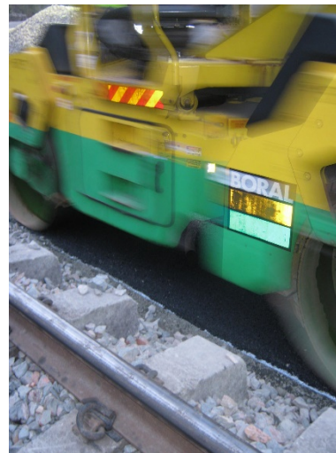
Figure 4: compaction of 2nd asphalt layer
