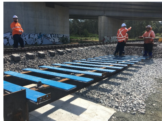
Figure 17: VTRAS support structure prior to ballast placing
