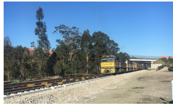
Figure 33: First coal train approaching IVES and high speed weigh bridge
