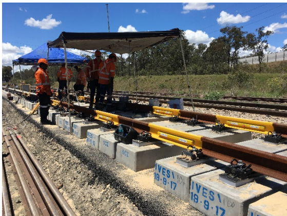
Figure 23: Completed IVES with customised spacing to suit the weighbridge transducer sets.
