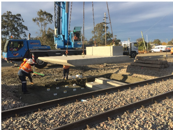
Figure 15: Placement of pre-cast abutment elements
