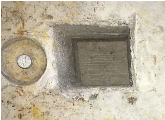
Figure 26: trial pocket with smooth walls
